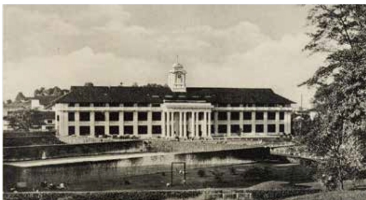
Singapore's first medical school was established within Singapore General Hospital in 1905
